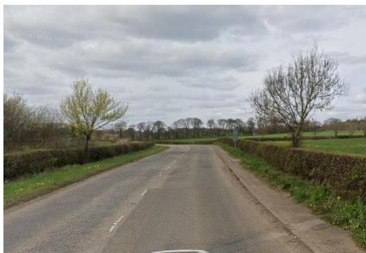
B9080 West of Kirkliston Fairly wide but some accesses and not consistently designed to modern standards.
